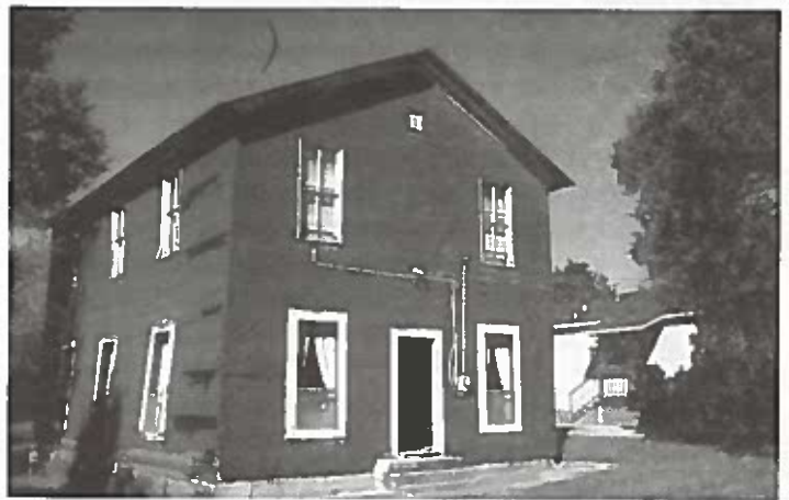
The Chickamauga Lodge #221 continues its significance in the African American community in Walker County. The preservation plan will provide a blueprint to make the facility available for community use while preserving space for Masonic meetings. Photo by Jeanne Cyriaque
